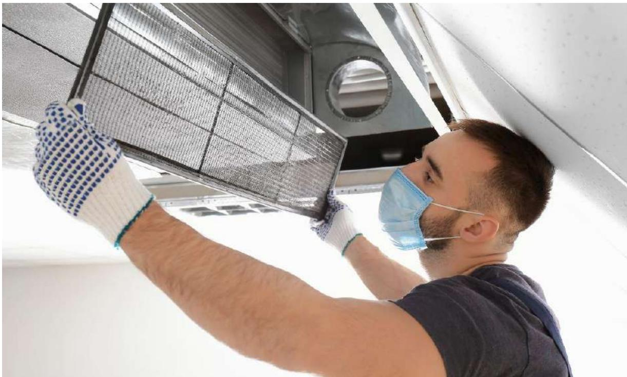
A functioning HVAC system is essential for maintaining acceptable indoor humidity levels, so it's important to keep up with HVAC maintenance. Clogged or dirty filters will impede airflow, reducing your HVAC's effectiveness. Clean or replace the furnace and air conditioner filters to restore airflow and reduce humidity levels inside the home.
