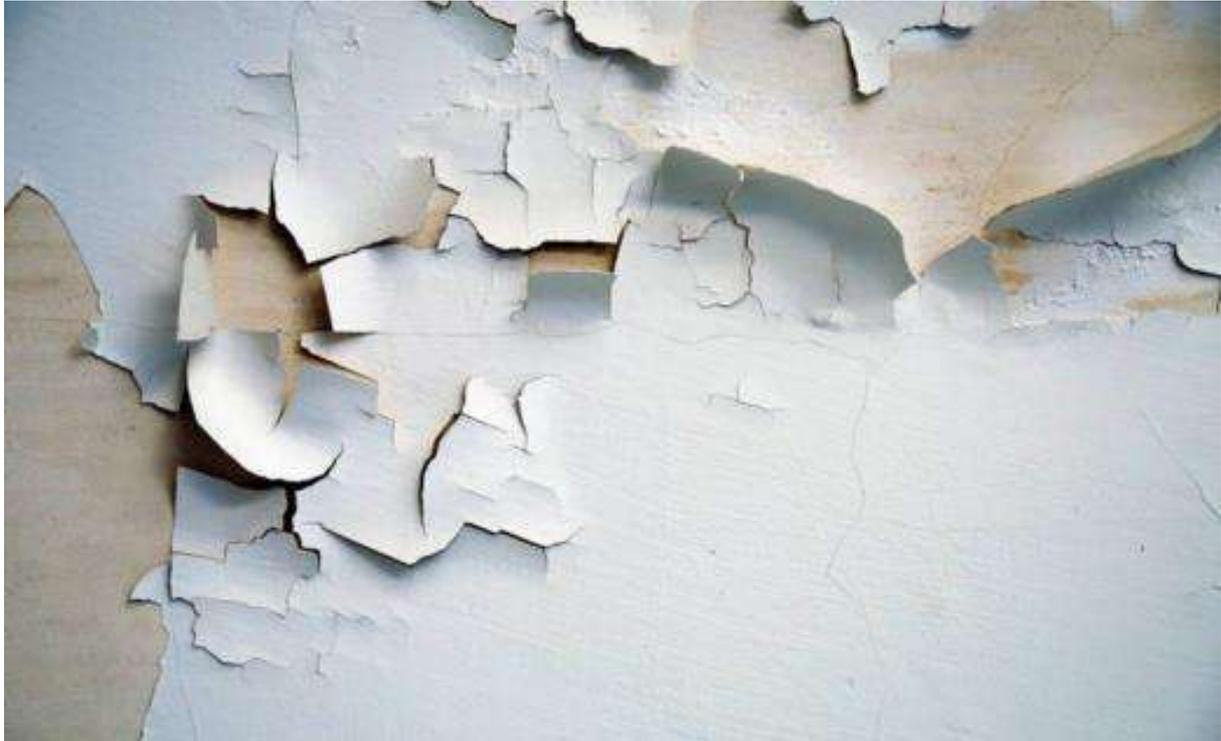
Water beads on the walls or any surface for prolonged periods can cause paint to start peeling.
